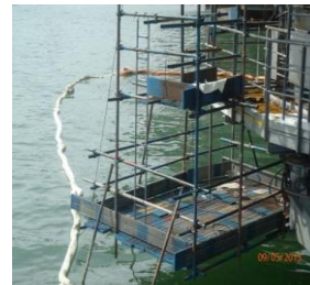
Containment Boom Deployed after Burst Hydraulic Line Caused Oil Spill
