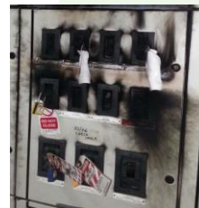
690V Electrical Switch Panel After Flash Fire
